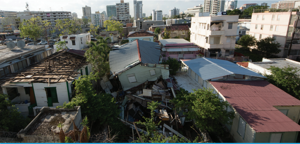
Homes in San Juan and across the island were heavily damaged by Hurricane Maria.
