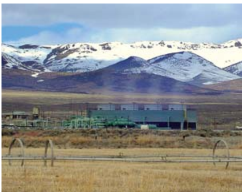
The Raft River Unit 1 began commercial operations in January 2008. PHOTO: Ormat Technologies, Inc.
