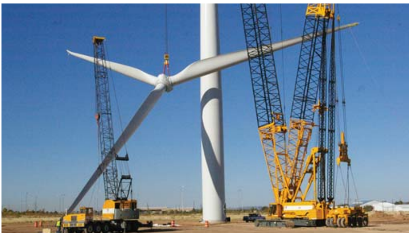
Wind turbine installation in Tucumcari, N.M. PHOTO: Mesalands Community College
