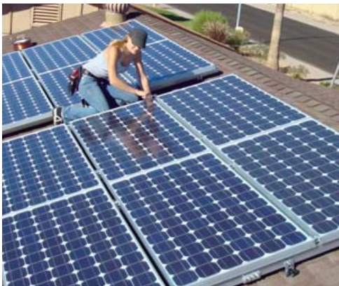
A worker installs a rooftop solar panel in Arizona.
