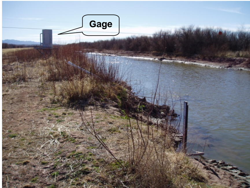
Figure 2 - Fort Quitman IBWC gage in the rectified channel at the upper end of the Forgotten Reach looking downstream.
