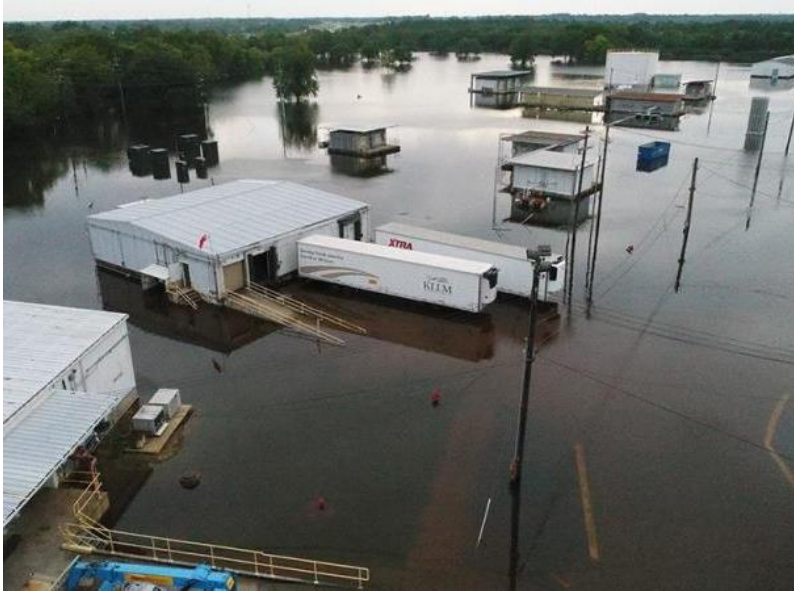
Flooded Arkema plant in Crosby, Texas. Image: Arkema
