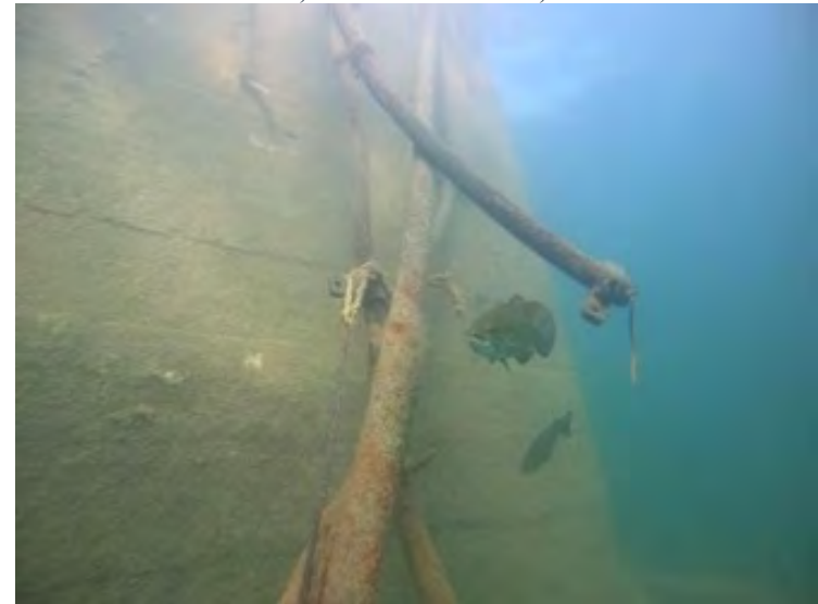
(D) Bare lead (upper-left). Cut end, near fish (mid-right). Site LP 4.1. August 2022, Lake Pend Oreille, ID.
