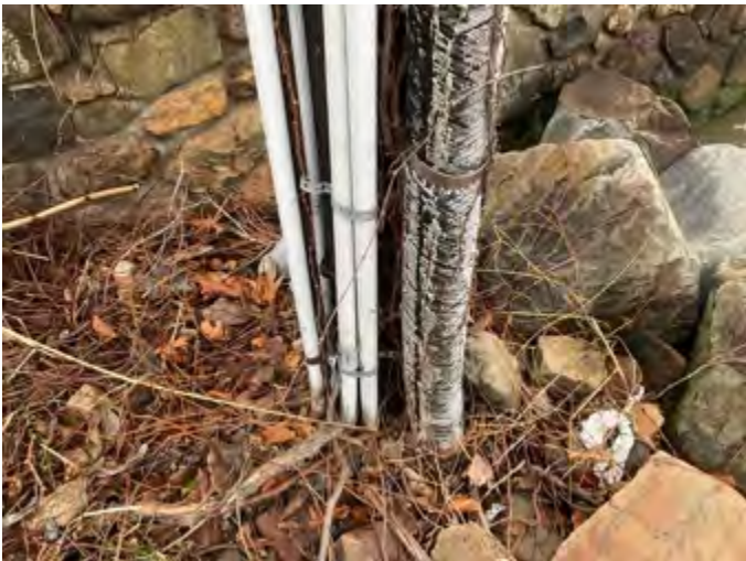
(I) Close up of abandoned 5" lead sheathed cable along the Hudson River. January 2023, Palisades, New York.
