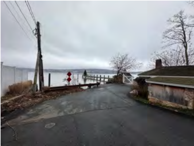
(H) Abandoned 5" lead sheathed cable along the Hudson River. January 2023, Palisades, New York.
