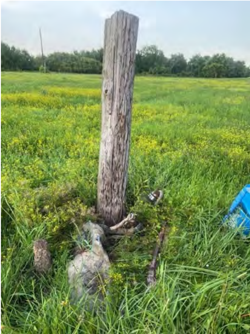
Figure 9 Photos. Louisiana continued. Damaged and abandoned leaded splice box and collection of five lead sheathed cables. MISS 12.3. June 2022, Donaldsonville, Louisiana.
