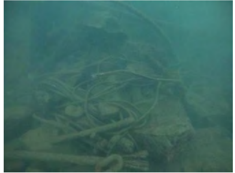
(F) Lead sheathed cables abandoned and coiled below the surface. Site LP 4.1. August 2022, Lake Pend Oreille, ID.
