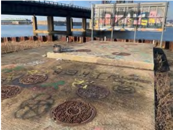
(A) Large vault with eight Bell Systems manholes on the Hackensack River. Looking towards South Kearny. January 2023, West Side, New Jersey.
