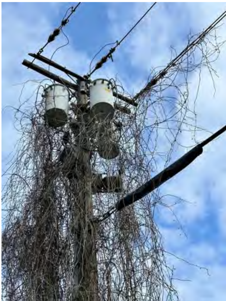
(F) “Squirrel Guard” tied around an exposed area of lead sheathed cable. Point of Interest: Newburgh 1. January 2023, Newbury, New York.
