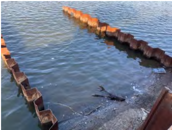
(B) Cable landing area covered with concrete. Area is below the sign in (D). January 2023, West Side, New Jersey.
