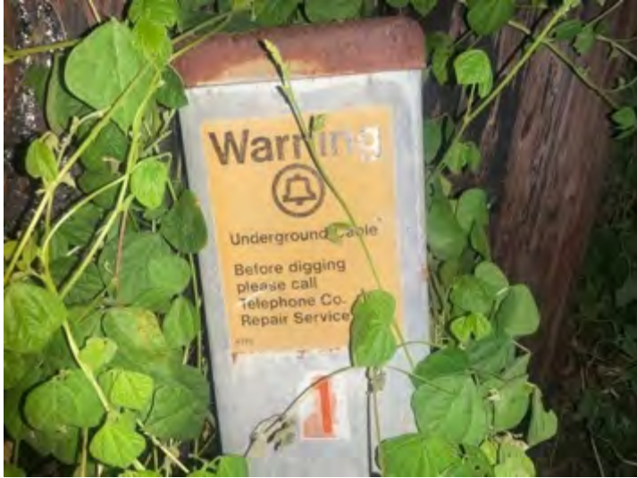
(A) Bell Systems sign for underground Telephone Cables. BL 2.1. Labadieville, Louisiana. June 2022.
