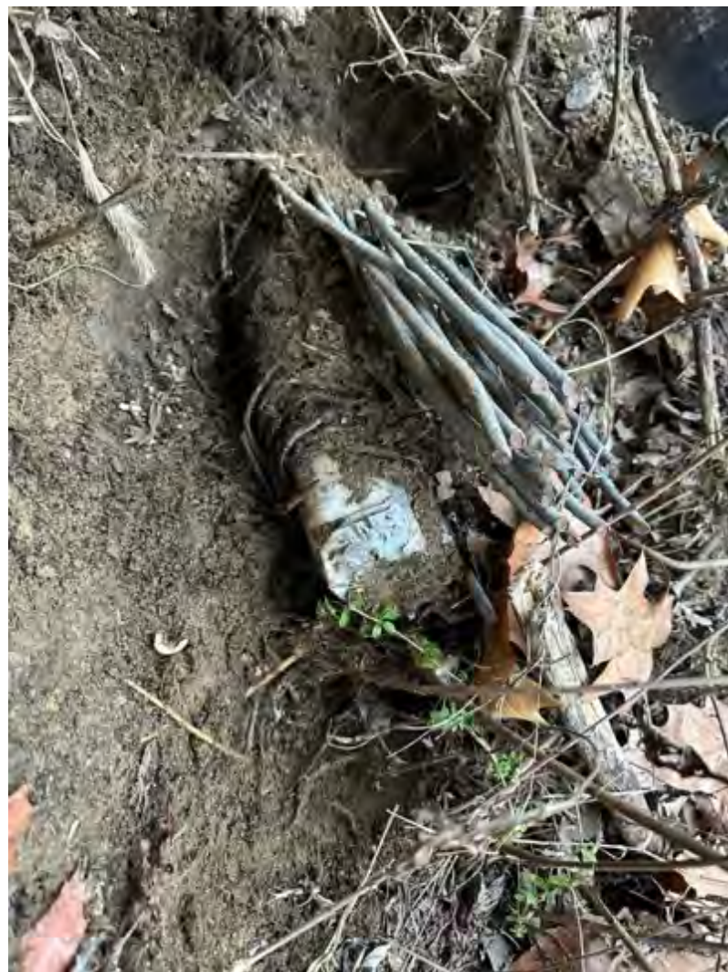
(E) Severed cable and steel wire at the base of an old telephone pole, across from those shown in (D). Point if Interest: Hudson 3.4. January 2023. Highland, New York.
