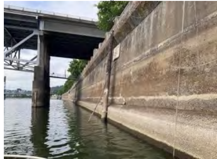
(D) Smaller lead sheathed cable below Western Union Telecom Co. Sign. WR 3. August 2022, Portland, Oregon.
