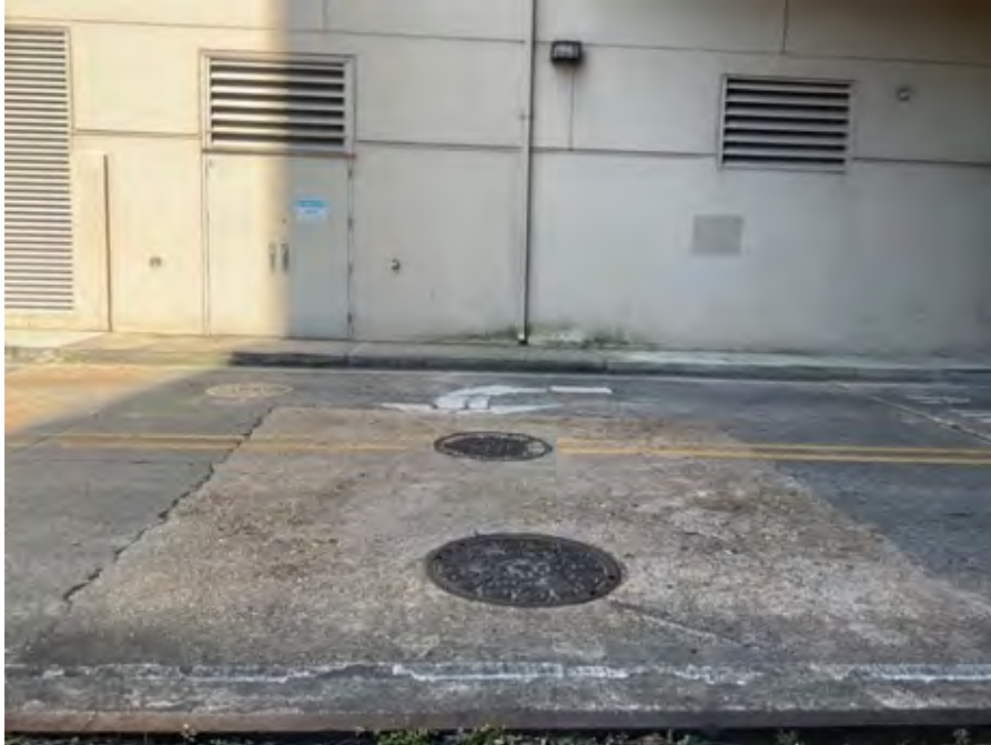
(I) New Orleans, LA. MISS 2.1 with Bell Systems manholes, vault, and Utility Building. This is a likely hub and splice area for cables, both old and new. June 2022.
