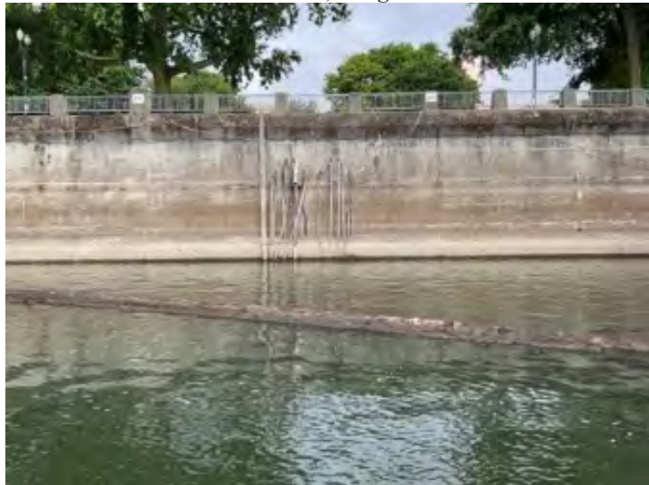
(B) Eleven cables near Maritime Museum and Waterfront Park. WR 2.2. August 2022, Portland, Oregon.
