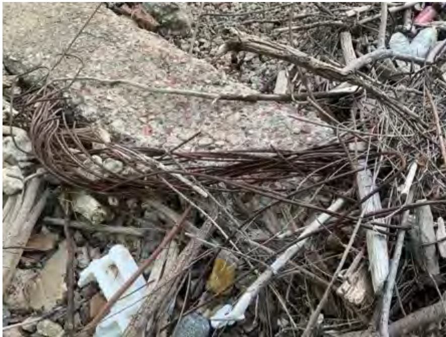
(L) New Orleans, LA. MISS 3.1. Remnants of outer steel wire from a lead sheathed cable. Evidence that parts of the cable may have been scrapped for money. Locals told us that that was done to these cables.
