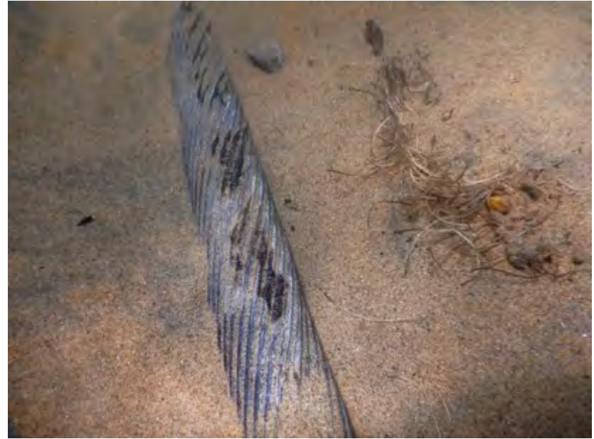
(H) 1920's lead sheathed cable resting on the lake bottom in Emerald Bay. May 2021, Emerald Bay - Lake Tahoe, California.
