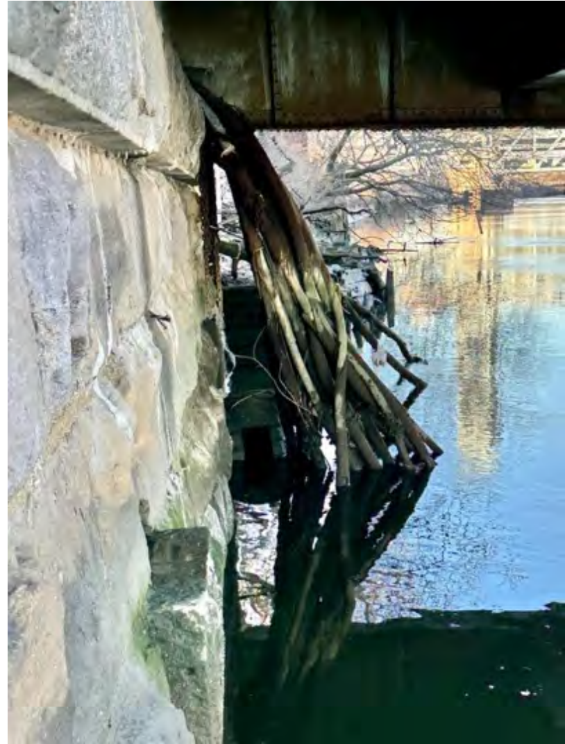
(I) Cable location with twenty lead sheathed cables underneath the Bridge Street Bridge (Harrison Ave.). Passaic 2.1 January 2023. Harrison/University Heights, New Jersey.
