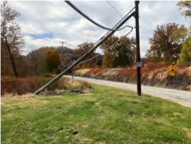
(E) CT8. Overhead lead sheathed cable running across a greenway and sidewalk. February 2023. Coal Center, Pennsylvania.
