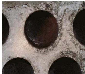
Clean boiler tubes provide optimal heat transfer.
